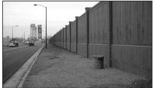
Exhibit 1. Noise Wall Isolating the Residential area from the New Roadway
